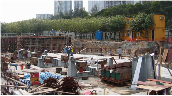
Figure 1. Cradle system supporting the Fireboat Alexander Grantham .
